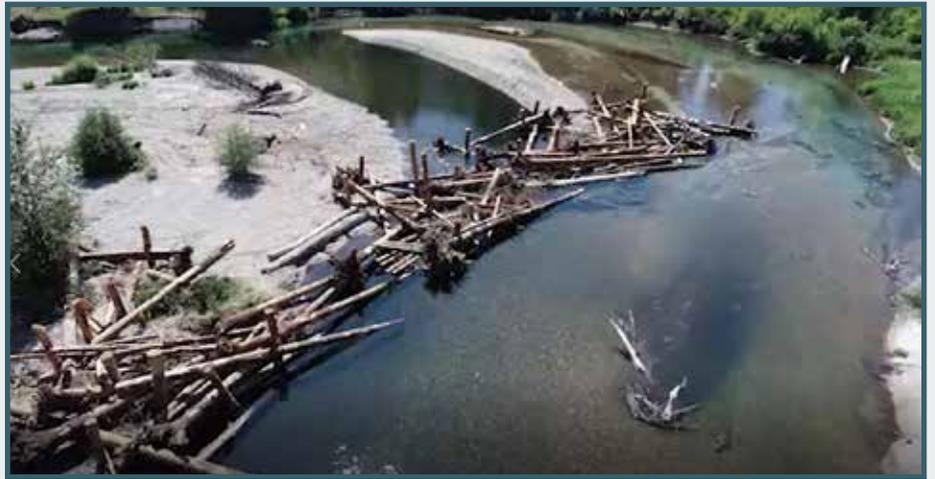
Some of the wood structures are placed to divert or push the river out onto the floodplain and side channels where plants, fish, and wildlife will benefit. This also helps with groundwater recharge and flood reduction.
